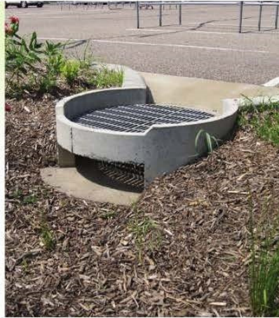
Many cities are using solutions, like this Rain Guardian inlet near Minneapolis to enhance bioretention function, speed up maintenance, and improve aesthetics. (Source: Rain Guardian)
