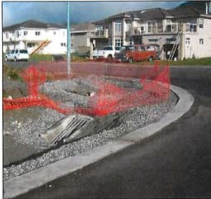
Figure 13: A low area with an outlet being used for sediment control at a construction site.
