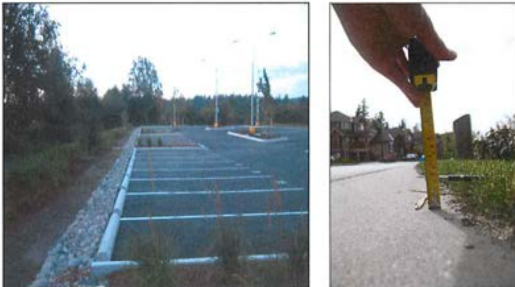
Figure 5: Non-erodible material should be used as a buffer between the asphalt and the rain garden (left photo). Do not use grass (right photo).
