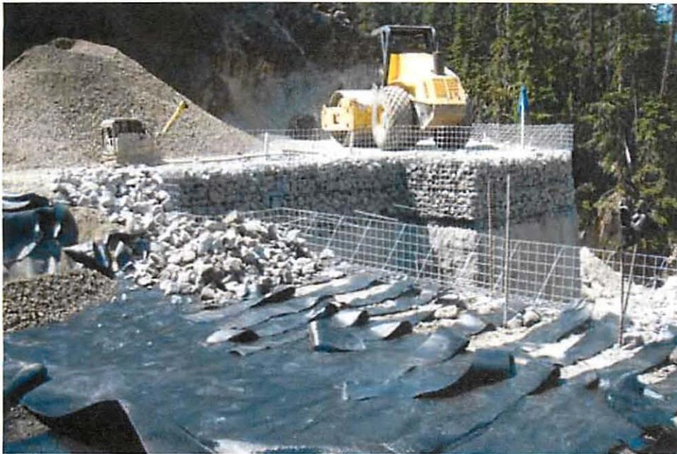
FIGURE 5 Irregular GRS wall alignment around left thrust block showing welded wire forms, backfill, geosynthetic reinforcement, and cobble facing zone. Photo: KWL
