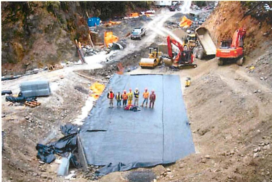
FIGURE 8 Geosynthetic fabric reinforcement rolled out parallel to wall face. Photo: KWL
