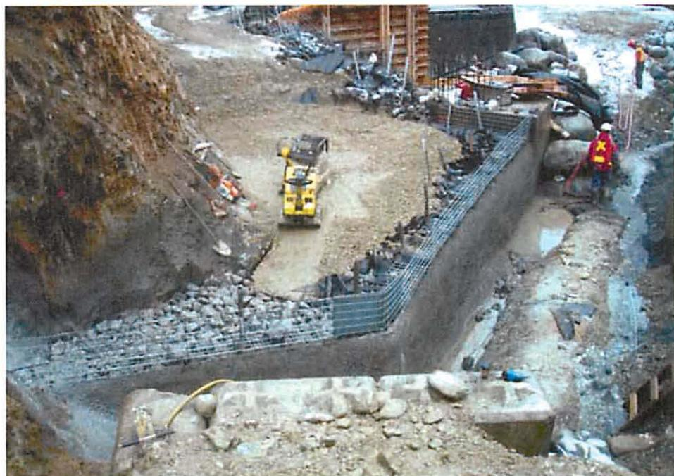
FIGURE 7 GRS tie-in to bedrock slope at upstream left abutment (note shotcrete facing). Photo: KWL
