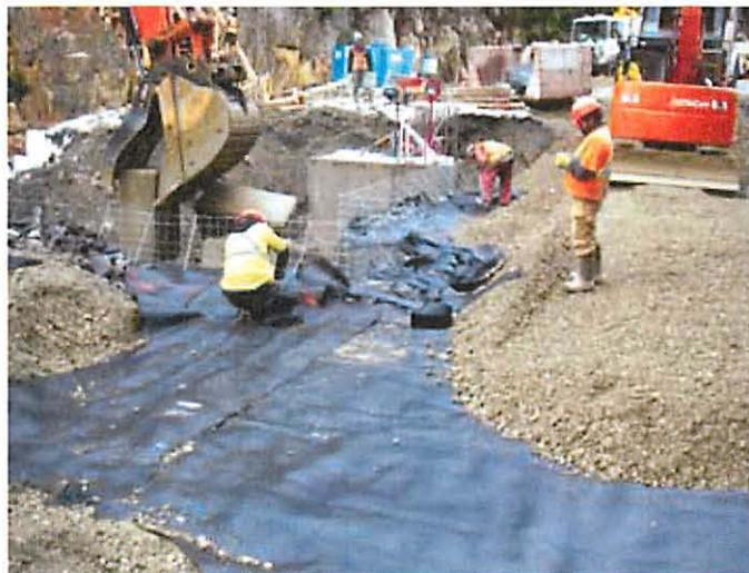
FIGURE 6 GRS construction around the left thrust block area (Note: no connection between reinforcement sections and reinforcement strips near face). Photo: BGC
